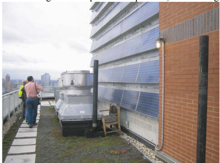
These solar panels would produce much more electricity if they were angled toward the sun, and were not shaded by rooftop equipment. As installed, they represent a colossal waste of perfectly good solar panels.
