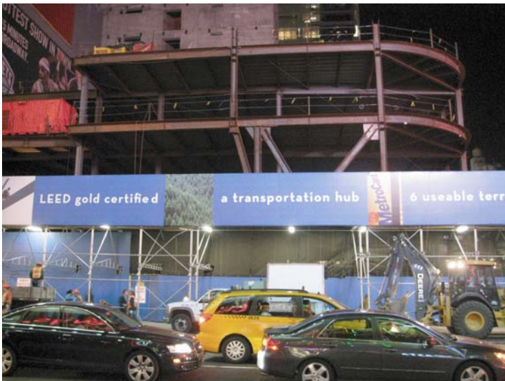
This sign is a daily reminder to every construction worker on the site that no matter how well they do their work, it will have no effect on the building’s environmentally friendly rating.
